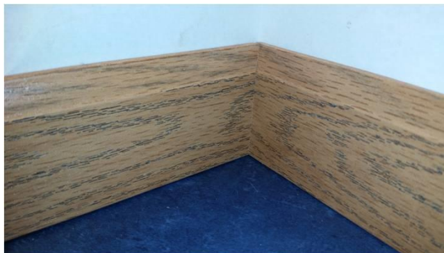
Figure 19-5. Finished Coped Joint.
