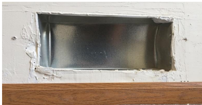
Figure 19-7. Sealing Plaster Gaps Around Cold Air Returns
