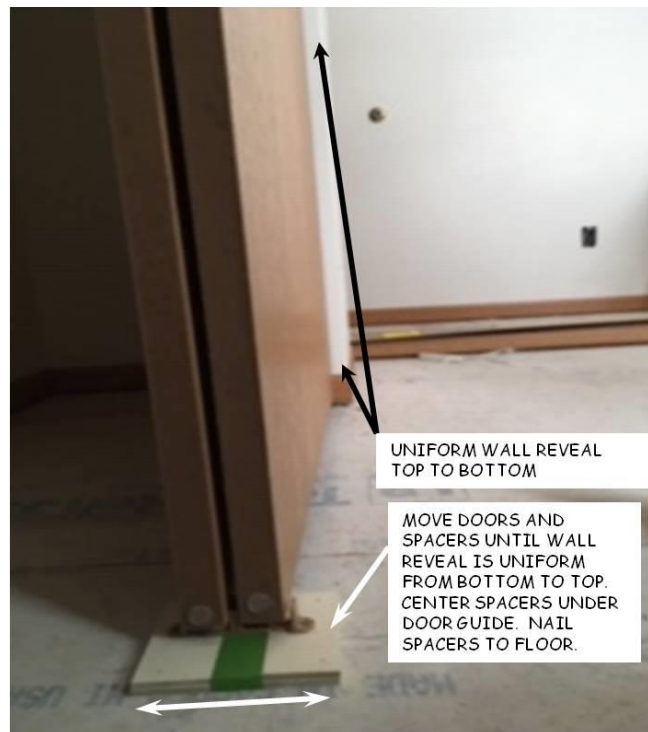
Figure 18-4. Shim Adjustment for Uniform Door Reveal.
