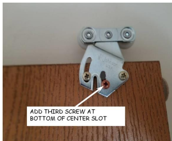
Figure 18-3. Closet Door Hanger with 3 rd Screw Installed.
