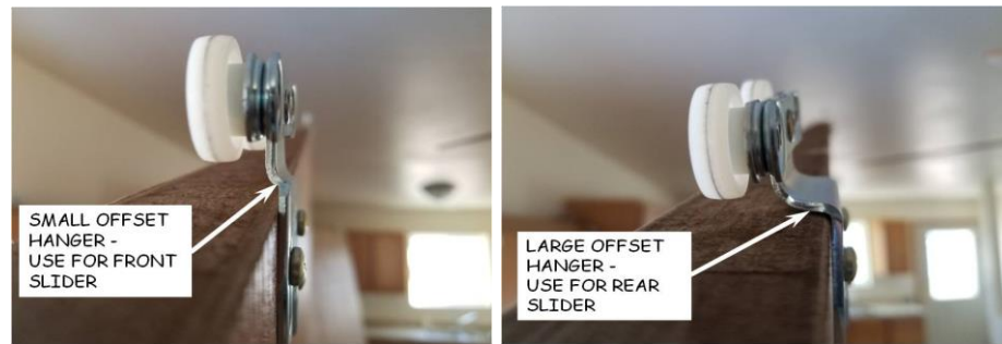
Figure 18-1. Sliding Door Hangers.
