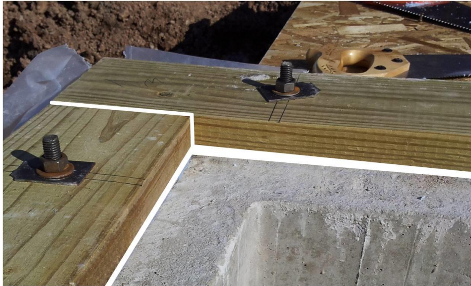
Figure 1-3. Sill Plate Installation.
